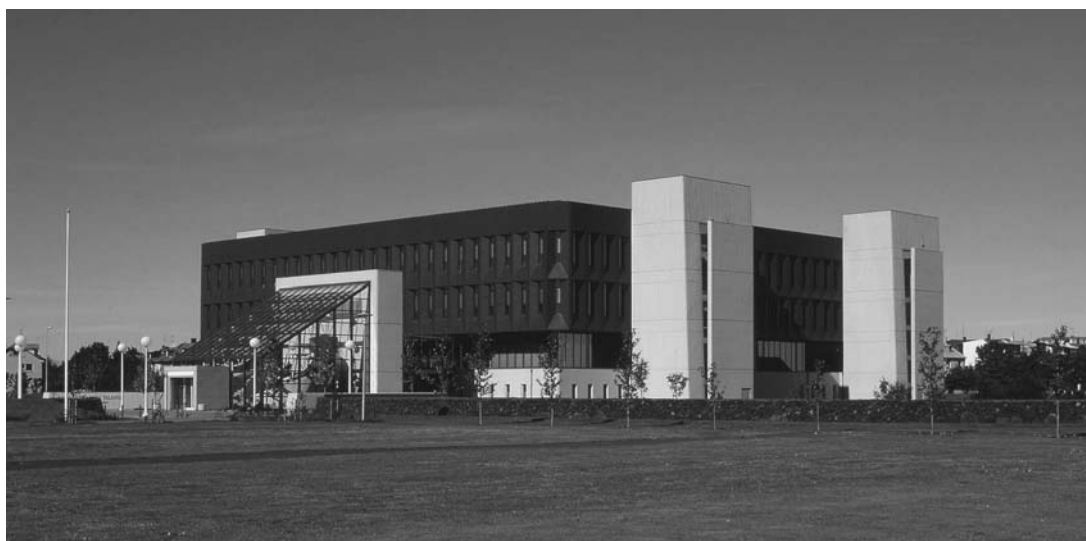
Figure 1. The National and University Library of Iceland: exterior view.
