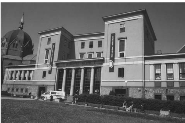
Figure 4. The Oslo Public Library. Deichmansk Bibliotek. Main building. Photo: Chris Erichsen.
